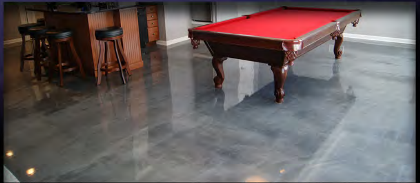
4. Clear Top Coat 3. Metallic Coat 2. Base Coat 1. Prepped Concrete
